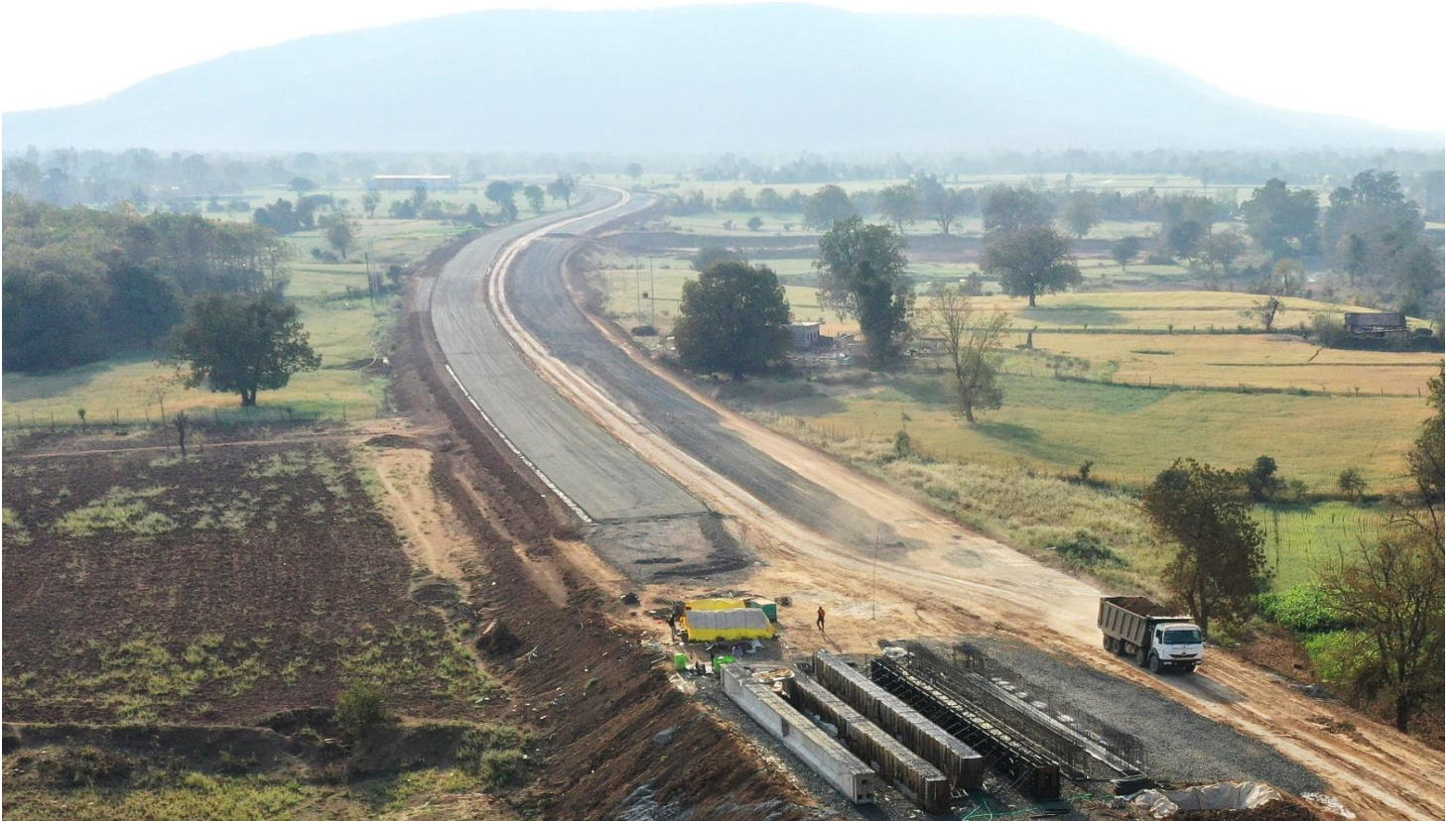
CTSB Work in progress
