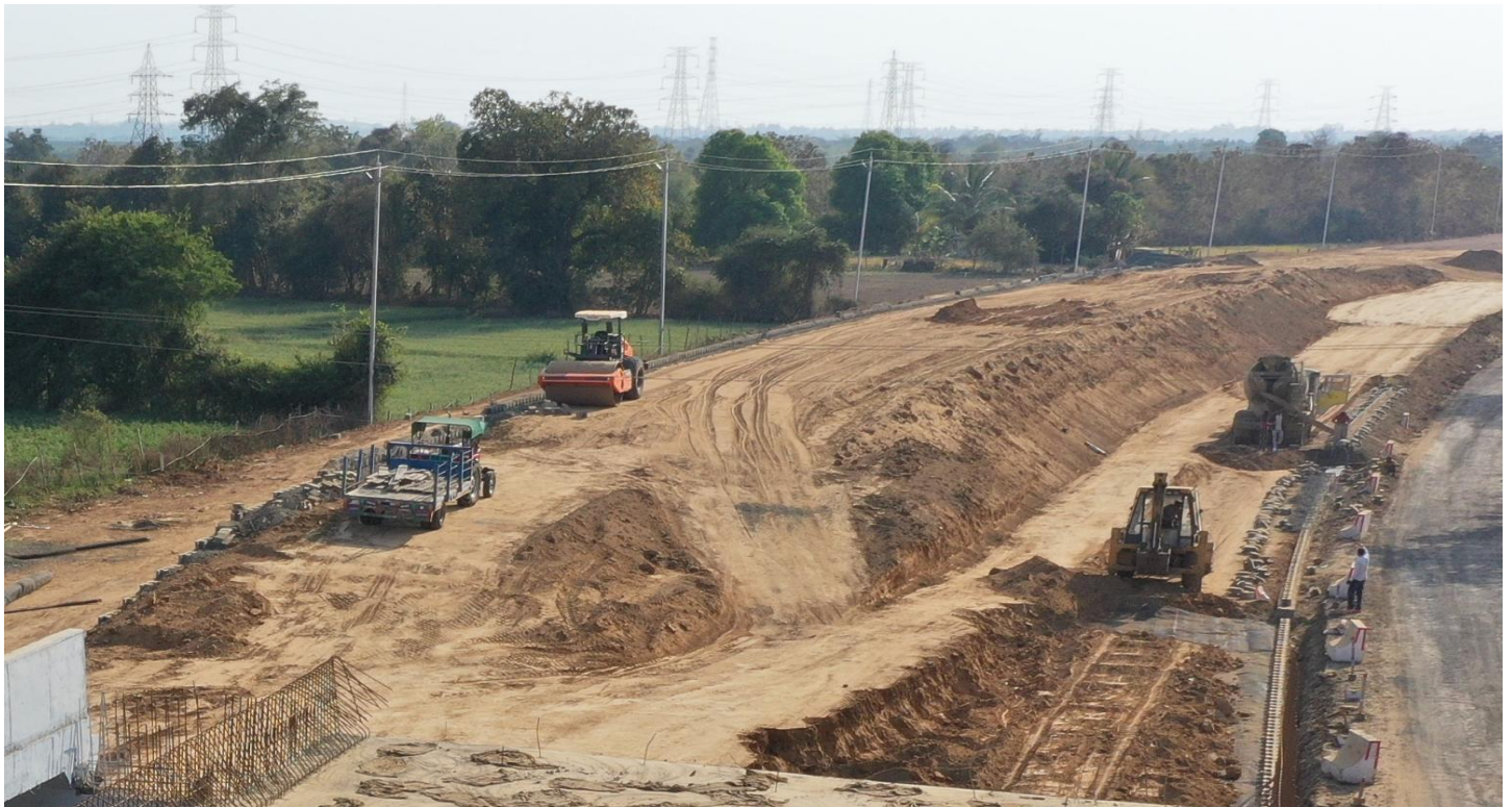
RE Wall Work in progress
