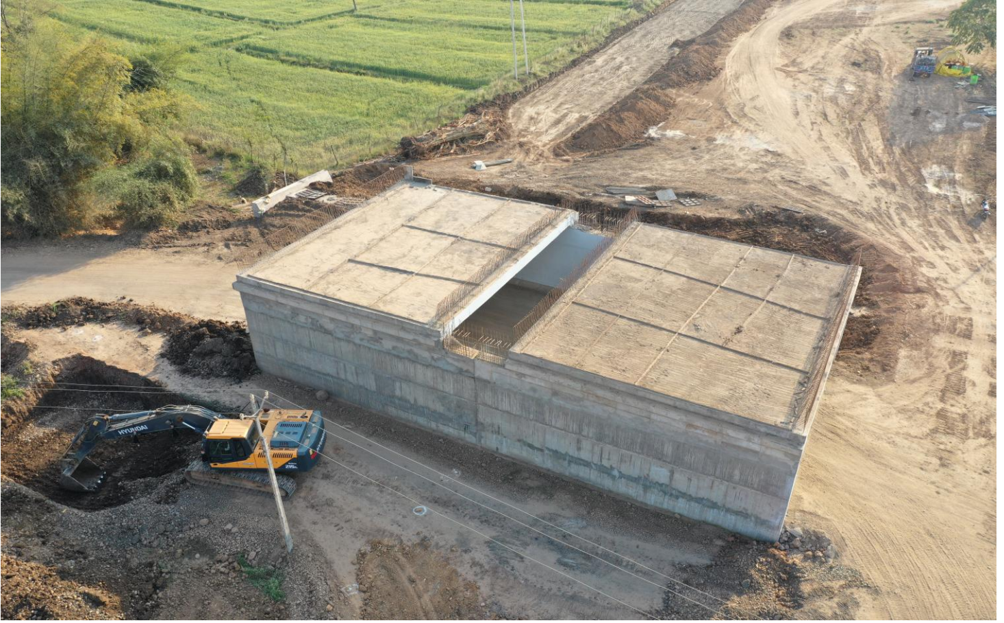
LVUP at 75+435 completed
