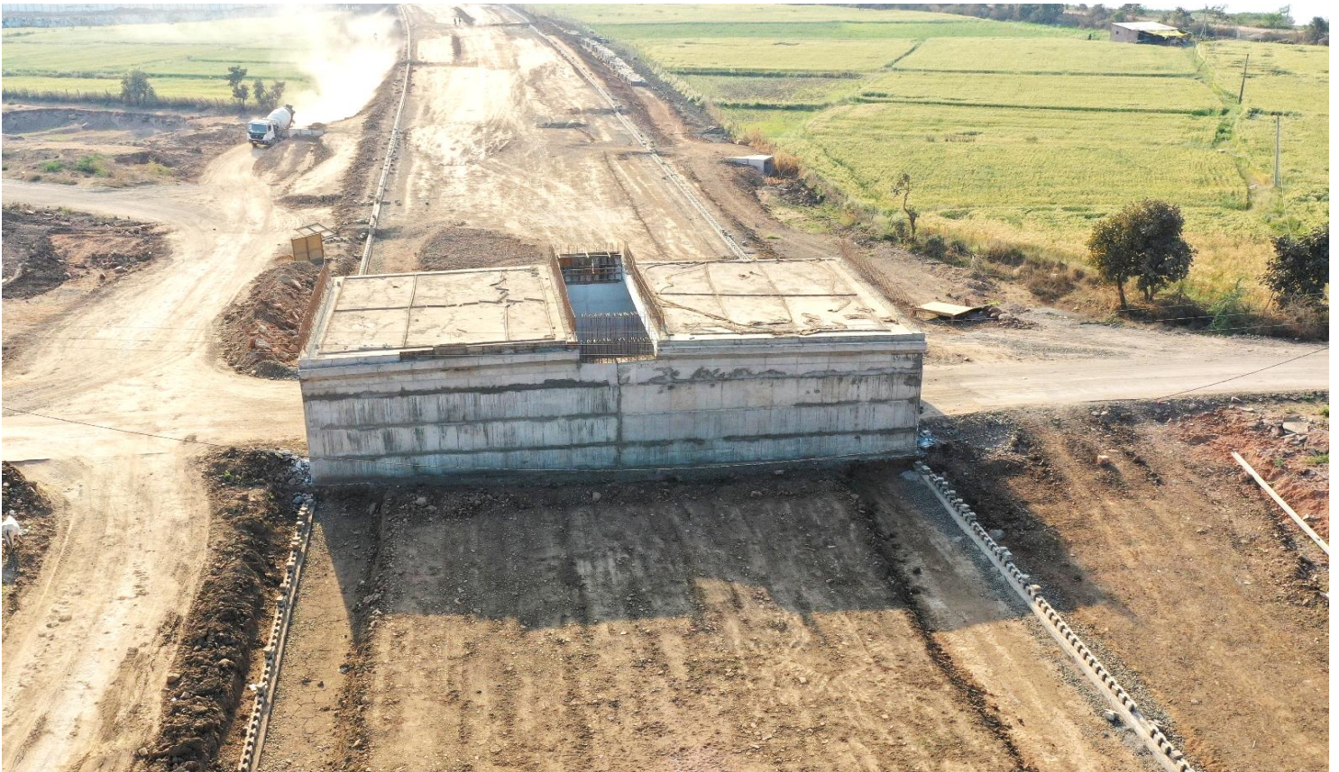
LVUP at 80+370 completed & RE Wall work in progress
