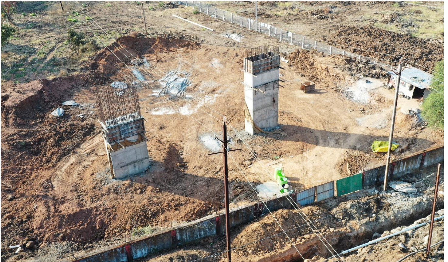
Work is in Progress at Km. 83+775 Flyover
