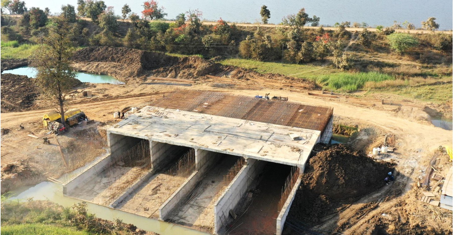
Work in progress of MNB at Km. 79+875
