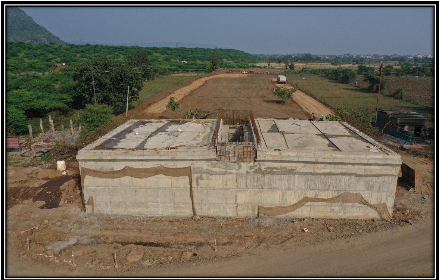
Work in Progress LVUP 80+372
