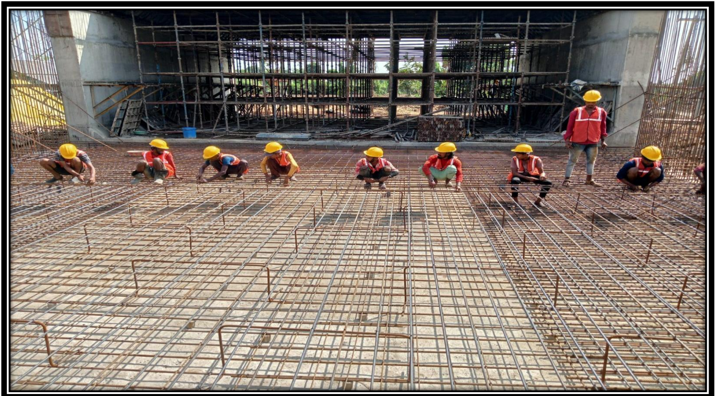
Reinforcement Fixing Work in progress of LVUP at Km. 92+428
