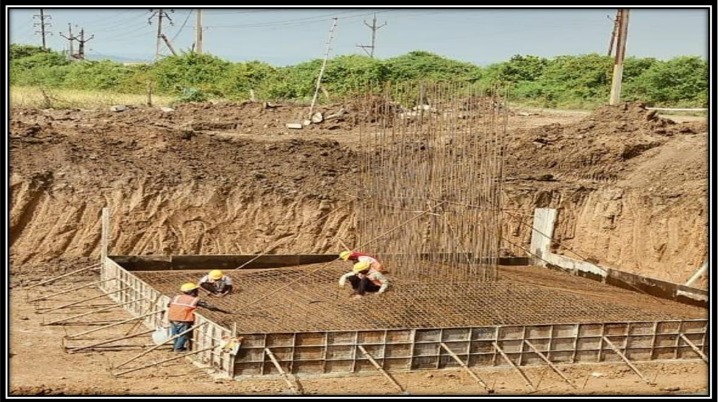
Reinforcement Work in progress of VUP at Km. 98+985
