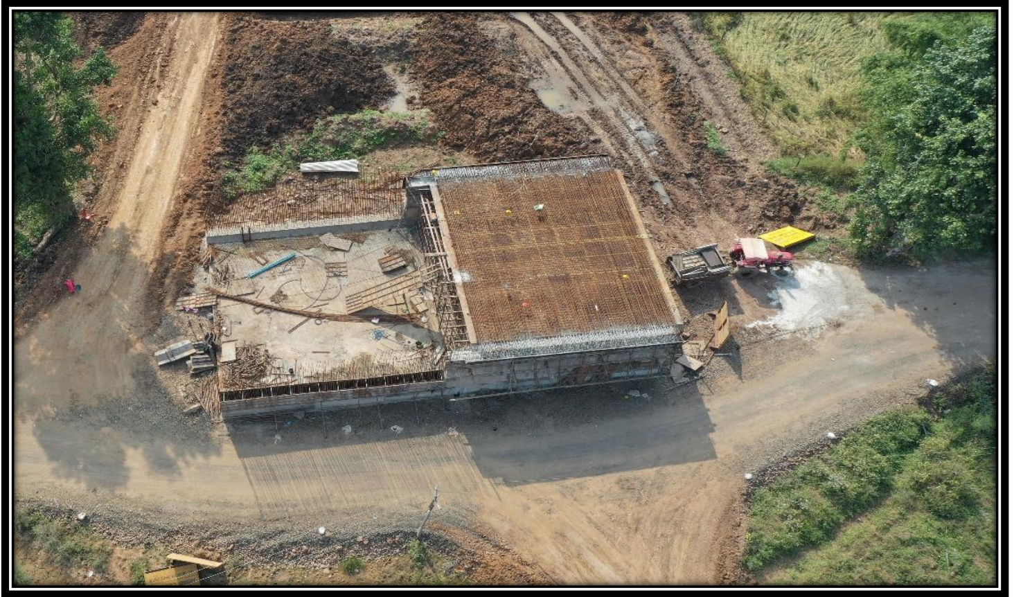
Reinforcement Fixing Work in progress of LVUP at Km. 92+428
