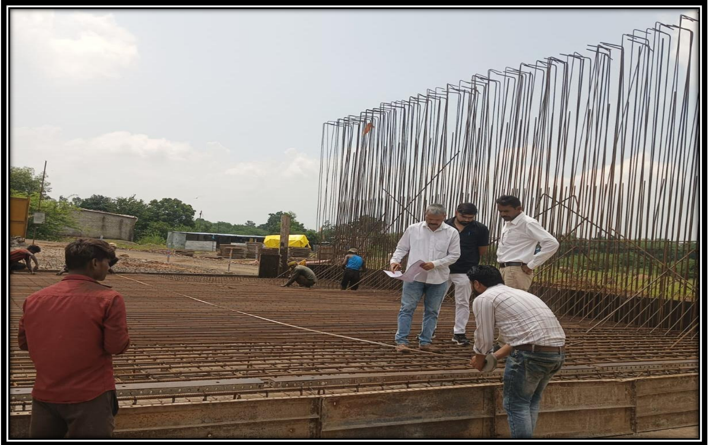
Work in progress of LVUP at Km. 80+372
