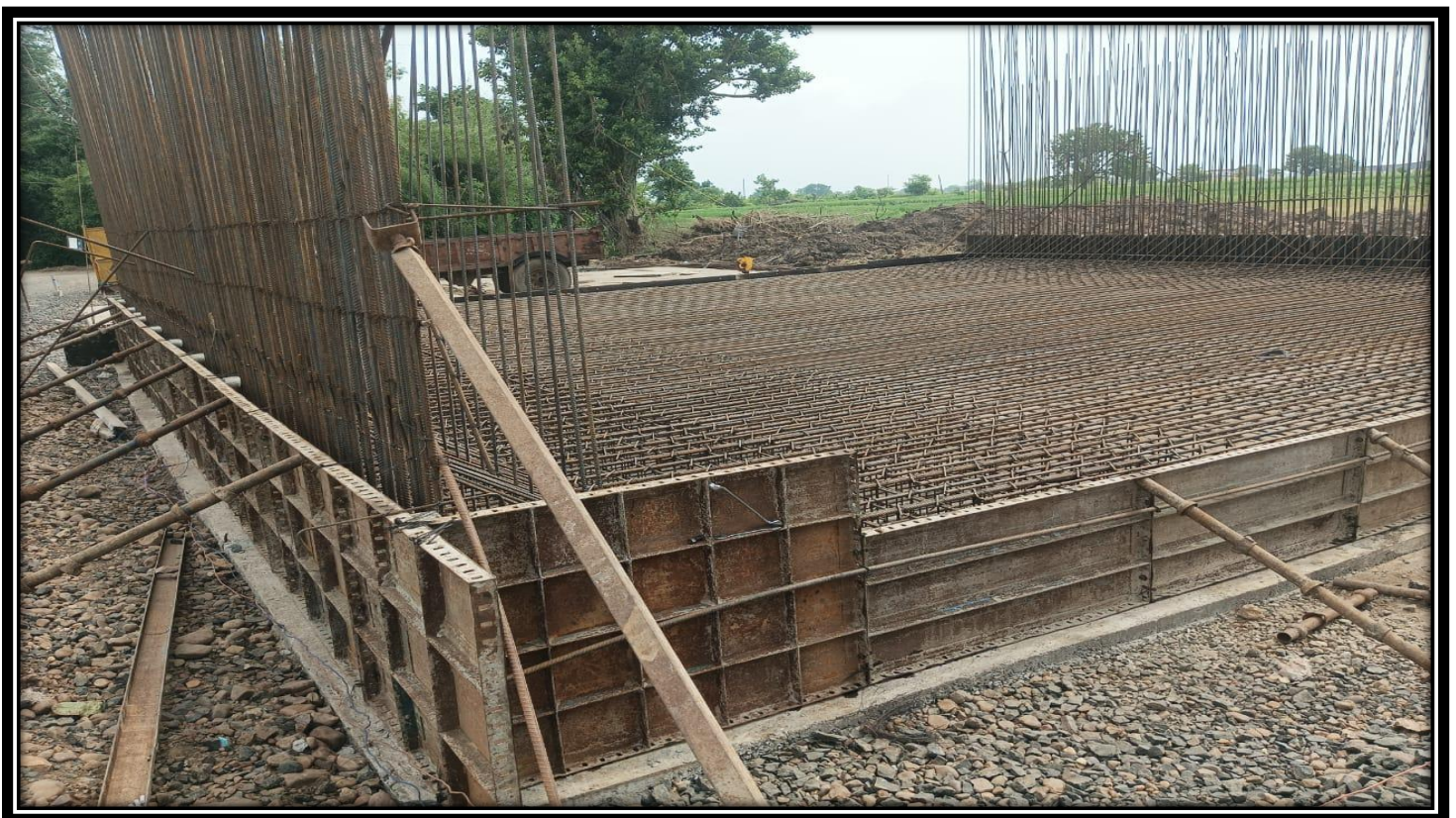
Work in progress of LVUP at Km. 75+426
