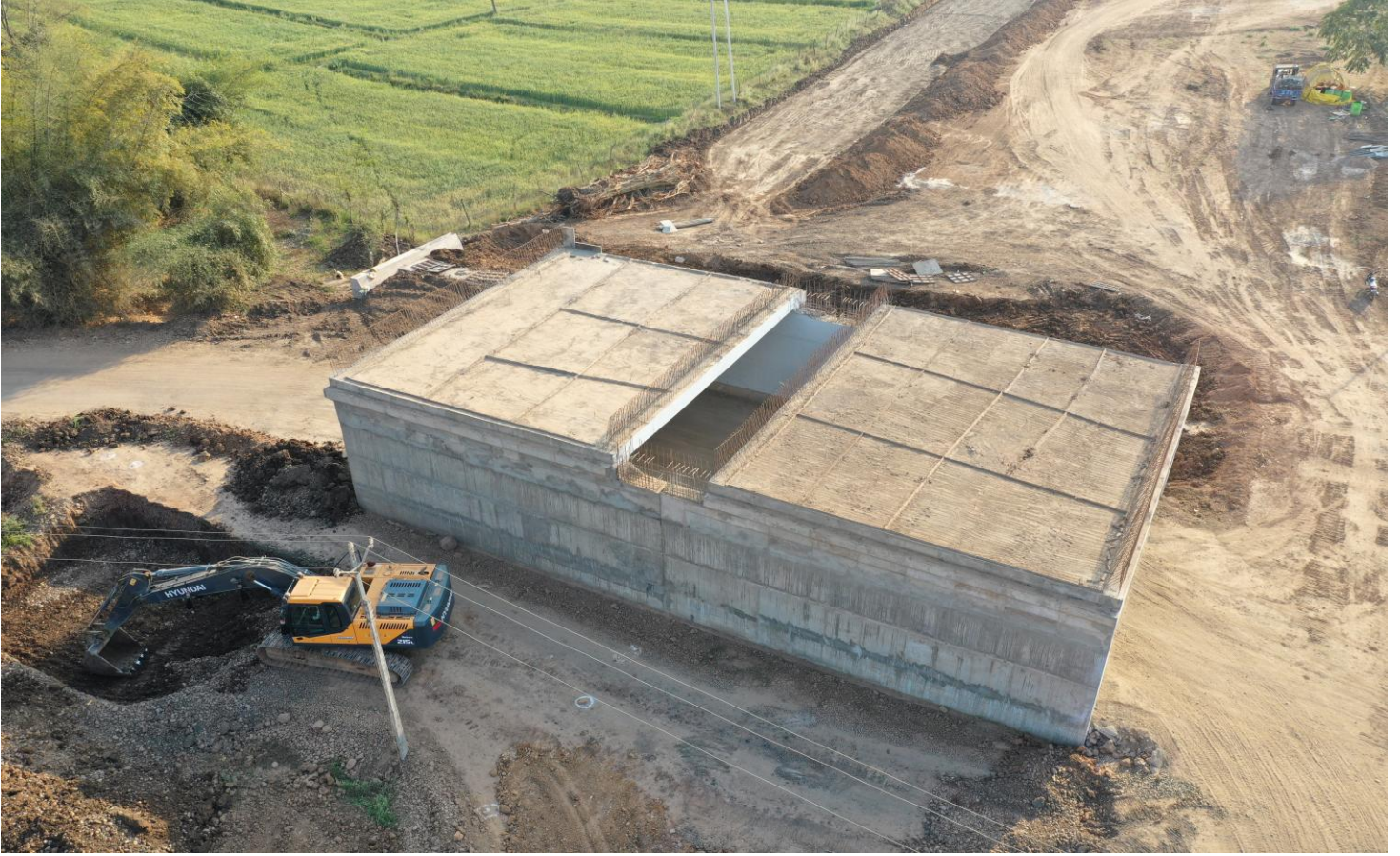
LVUP at 75+435 completed
