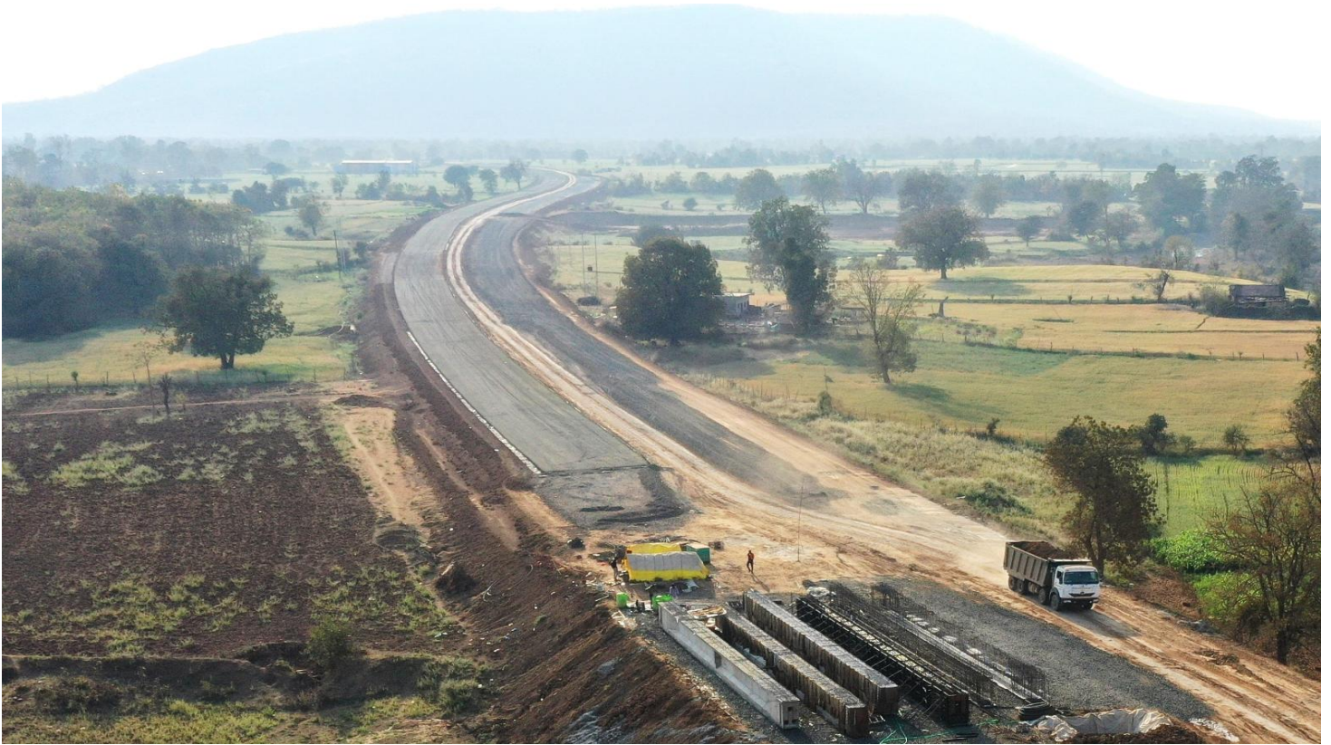
CTSB Work in progress
