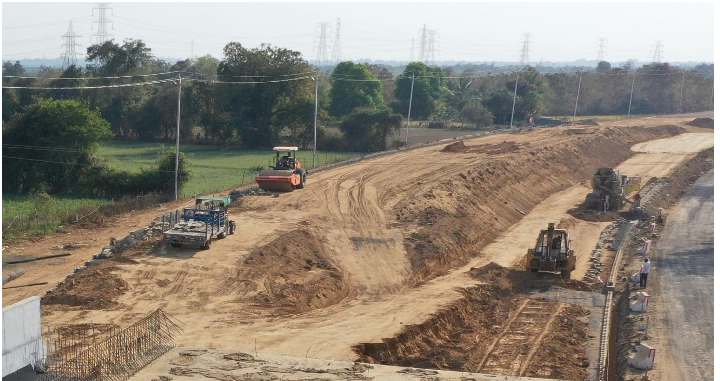
RE Wall Work in progress
