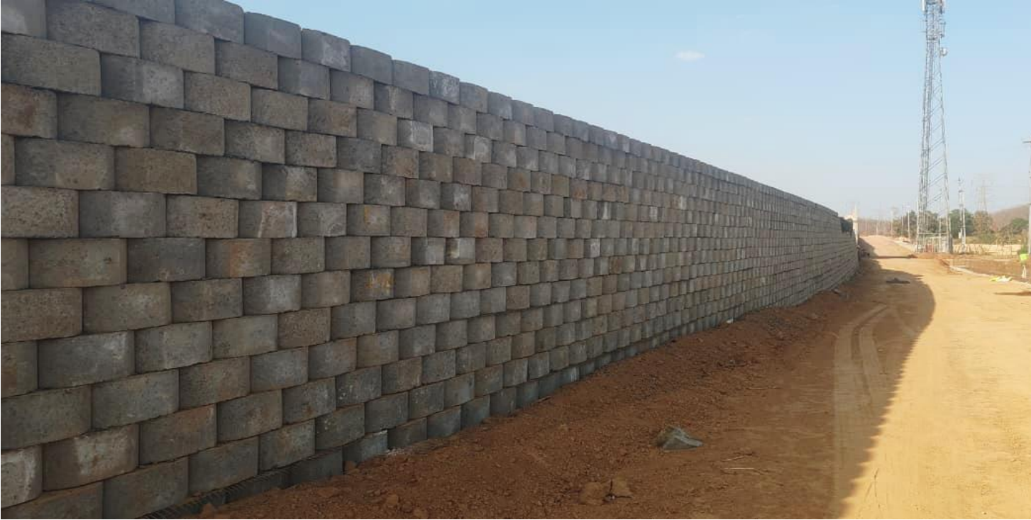
RE Wall work in progress
