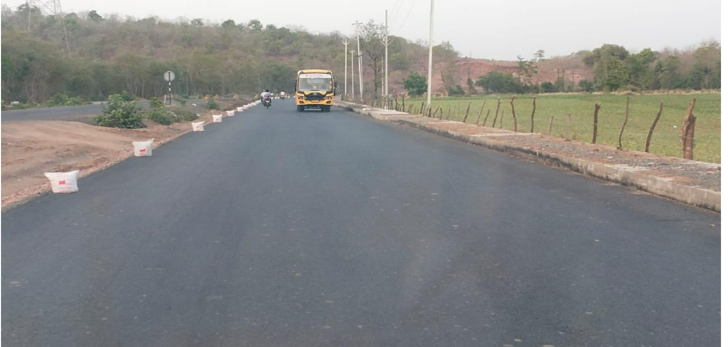
DBM Laying completed
