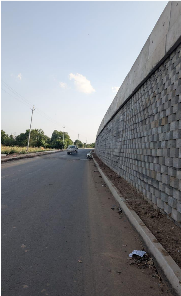
RE Wall work in progress @ 95+330
