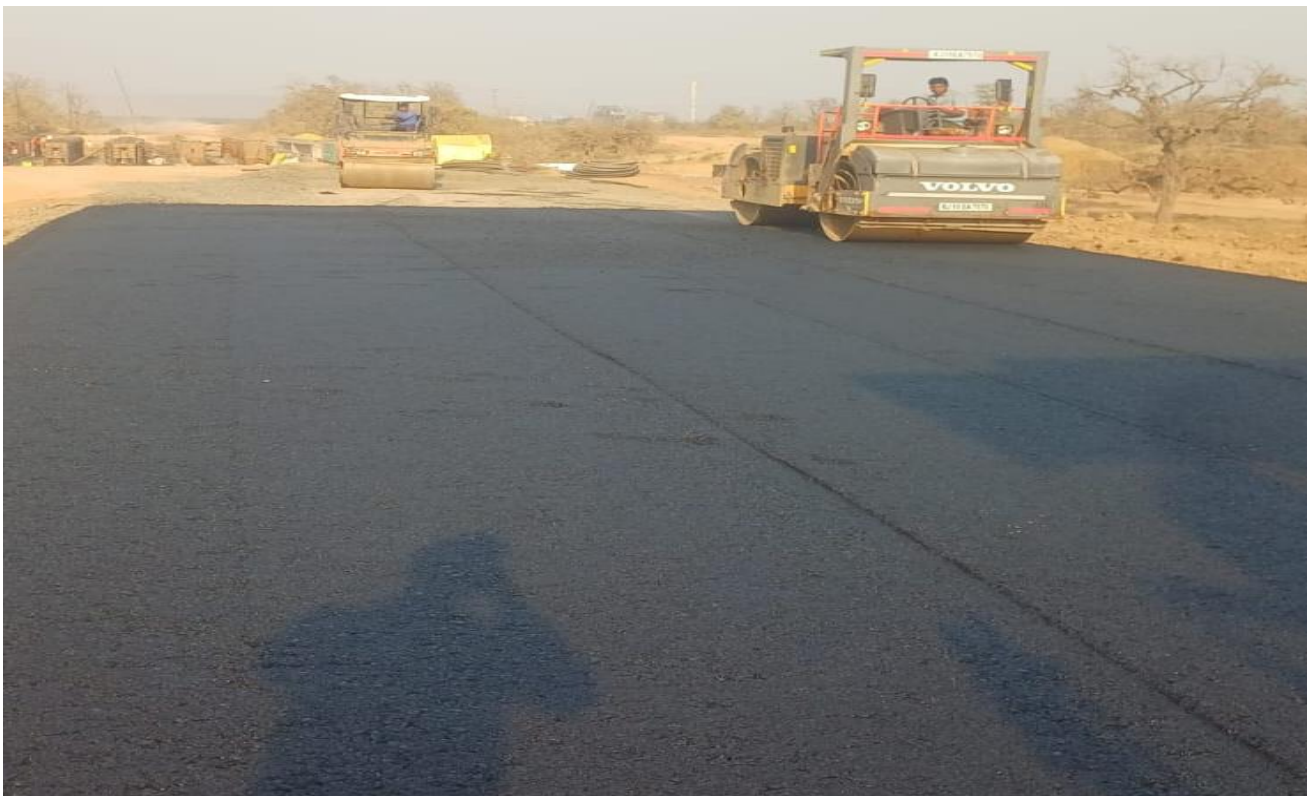
DBM Laying work in progress
