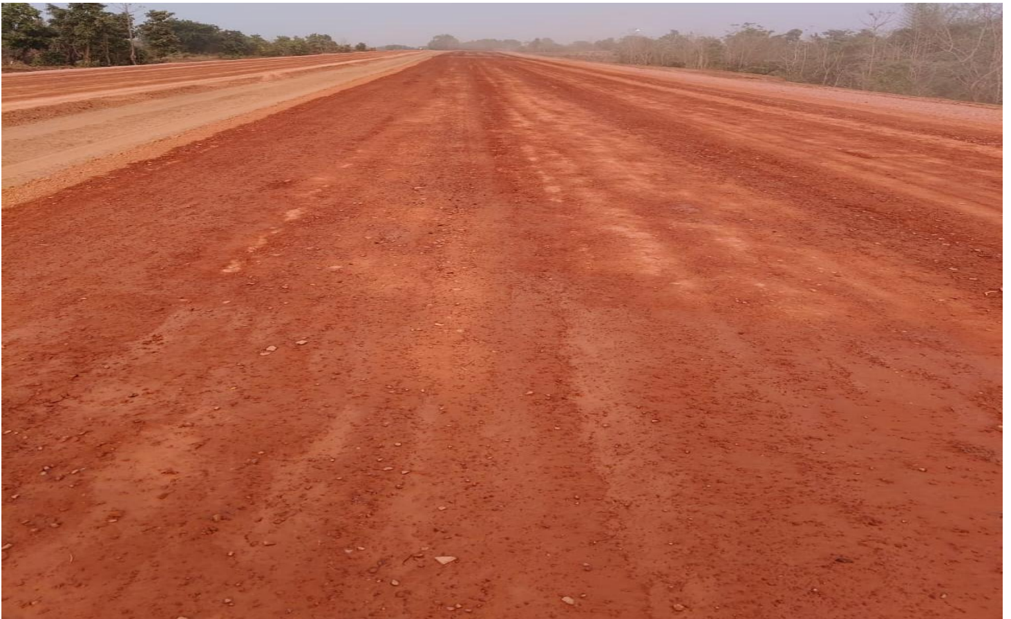
CTSB Curing Work in progress
