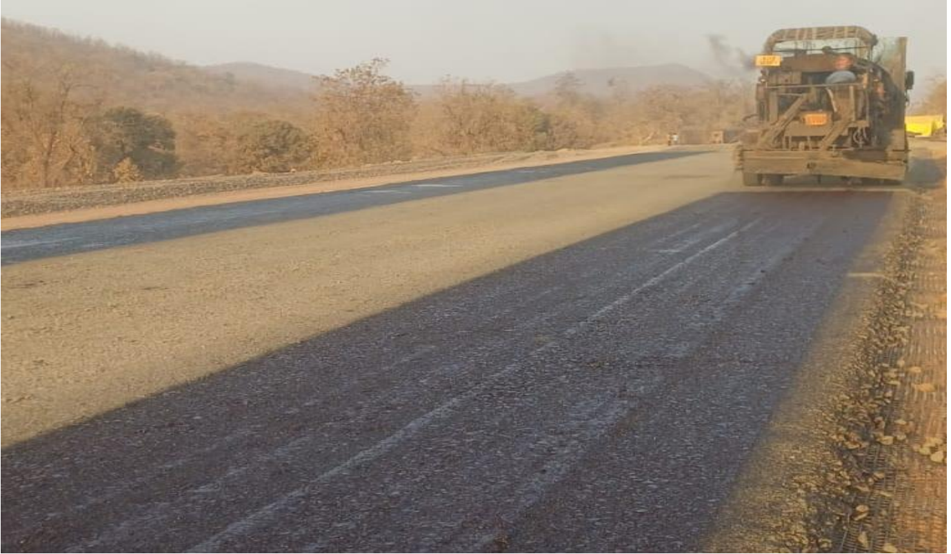
CTSB Curing Work in progress
